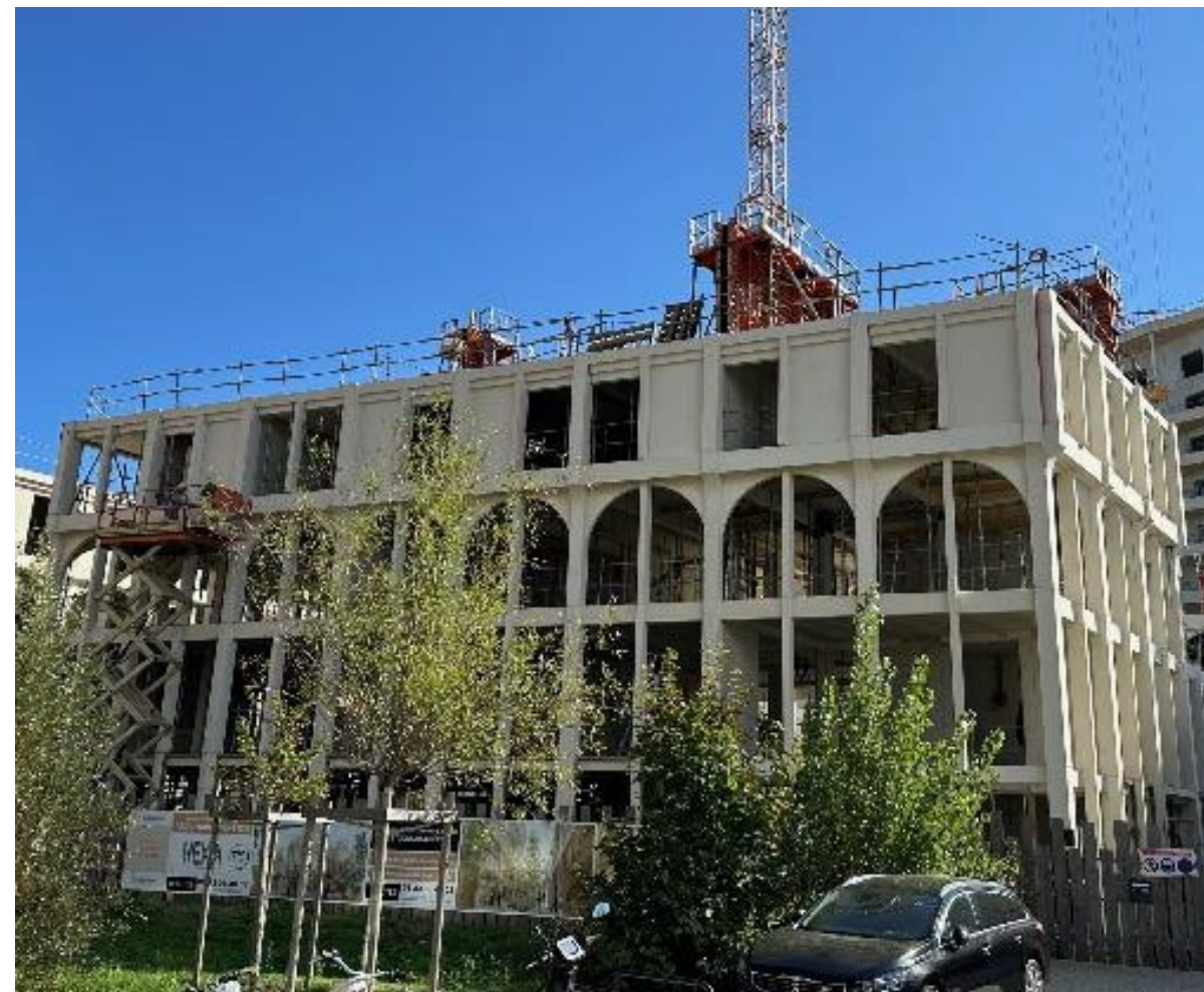
HEKA (Bordeaux) Construction de 95 logements mixtes
